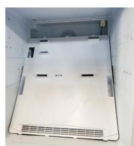
3. Remove the air duct cover
