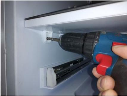
1. Remove the 2 screws at the bottom of the display partition
